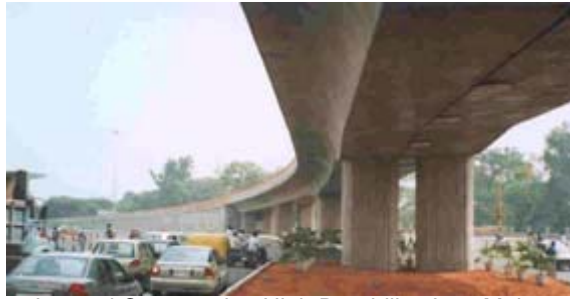
Fig.3: Kalkaji Flyover-Integral Construction High Durability, Low Maintenance, Increased Safety
