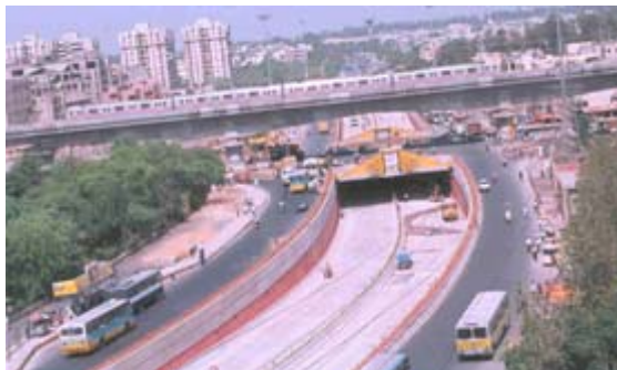
Fig.2: MRTS Viaduct & Underpass at Pitampura, Delhi
