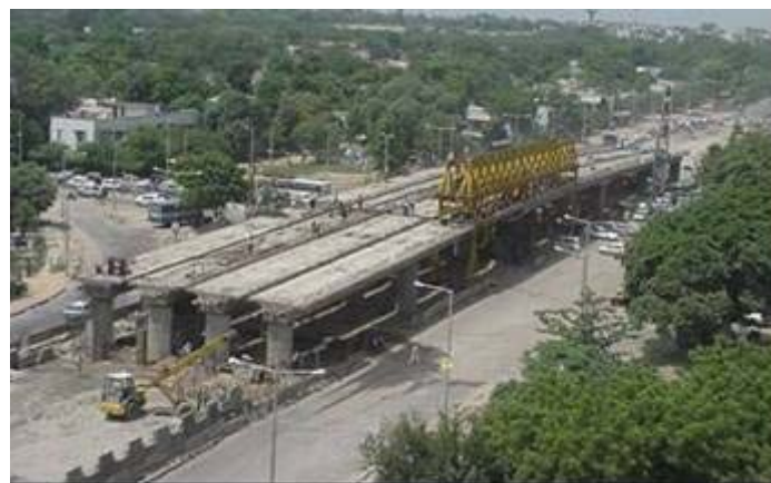
Fig.4: Erection of Various Stages Completed
