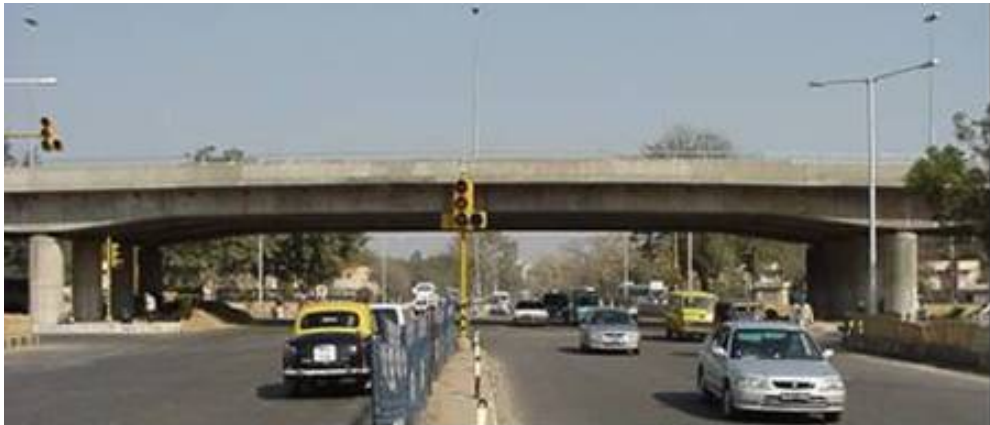
Fig.1: Main Span with Span/Depth Ratio of 27.6
