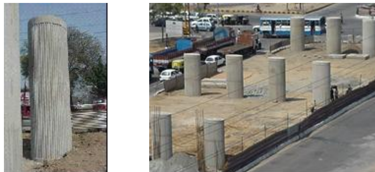
Fig.3: Elliptical Piers with Textured Surface
