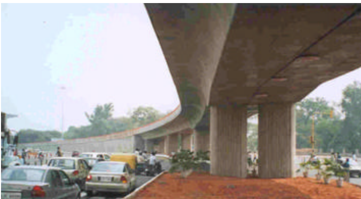
Kalkaji Flyover: Integral Construction High Durability, Low Maintenance, Increased Safety
