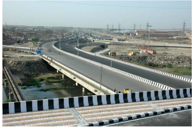
View from Busbay of Main Flyover
