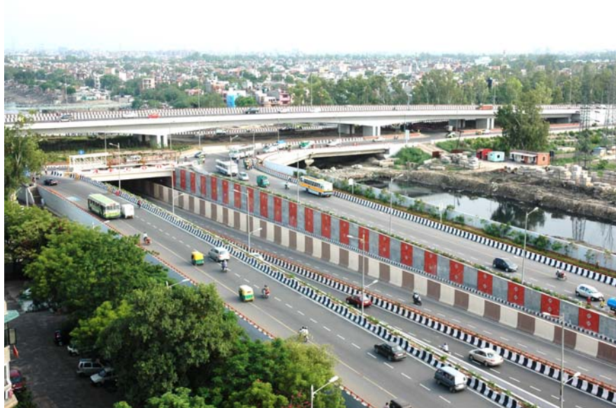
Fig.1 Three Level Grade Separator at Ghazipur Intersection on NH-24
