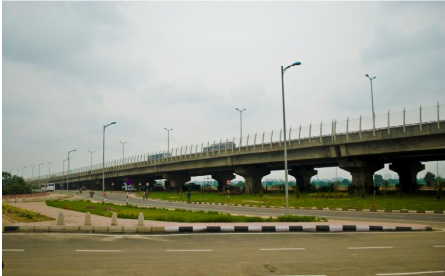
Fig.5 Flyover at Intersection of NH-24 and Bund Road near Commonwealth Games Village
