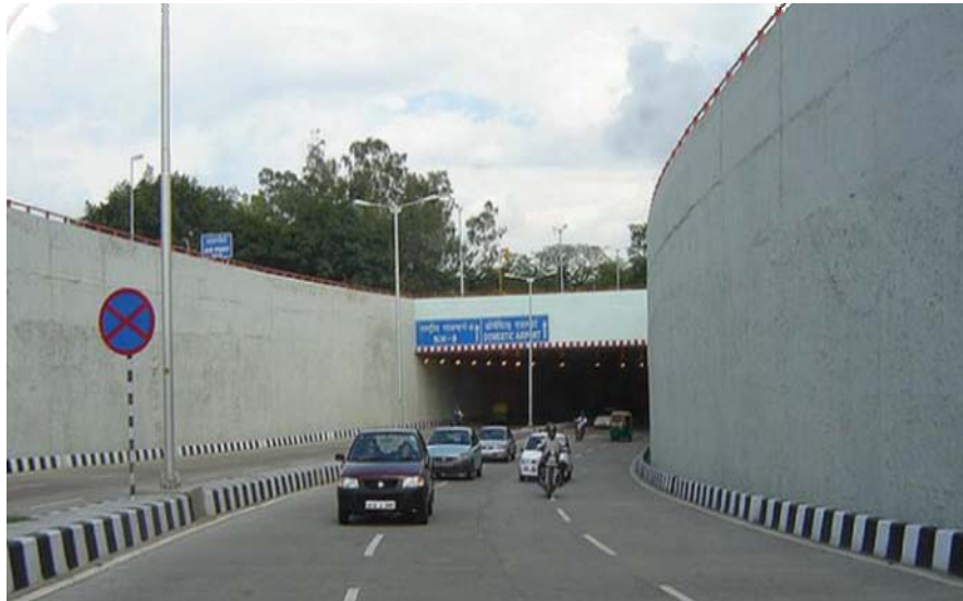
Fig.6 Underpass at Rotary near Domestic Airport Along Road Connecting to Dwarka
