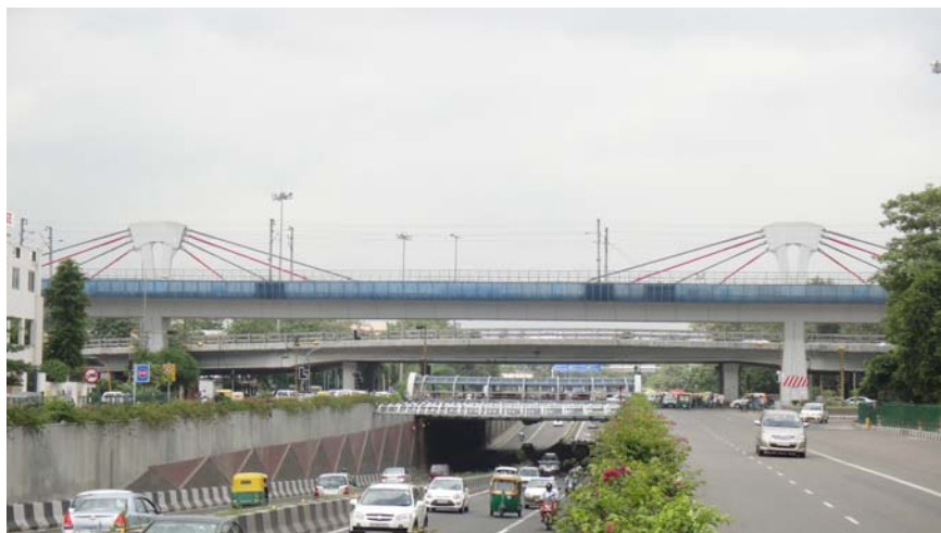
Fig.7 Extardosed Bridge at Moolchand Intersection for Delhi Metro
