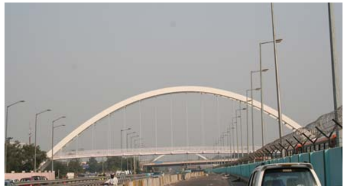
Figure 1. Photo Showing 80m Span Bridge (90m Span Bridge in the Background)
